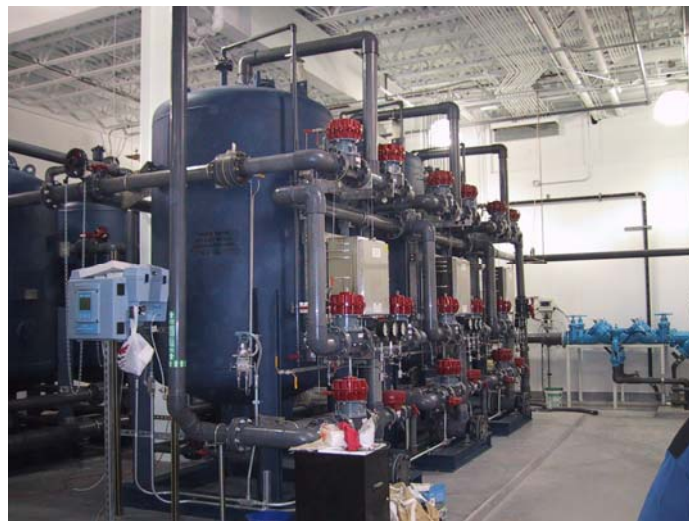
Figure 3. Typical Multi Media Installation
